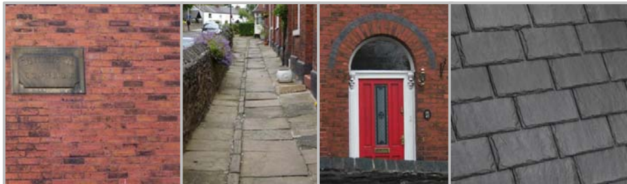
Traditional high quality materials: Red brick with blue detailing along with grey slate roofs and sandstone set walkways, boundary treatments, sills and headers represent historic local vernacular.
